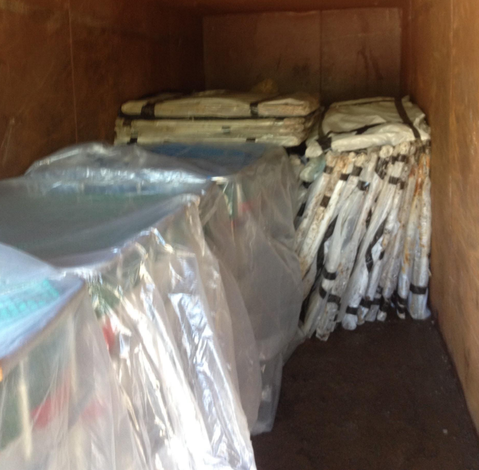
Asbestos box- separate from unsorted C&D waste
